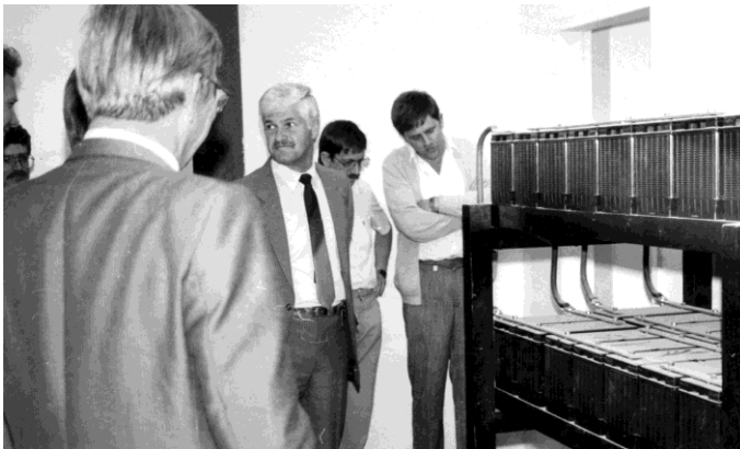
Figure 26 The batteries for emergency power in the new machine room. (Source: Photo collection of Mrs AD Mans)
