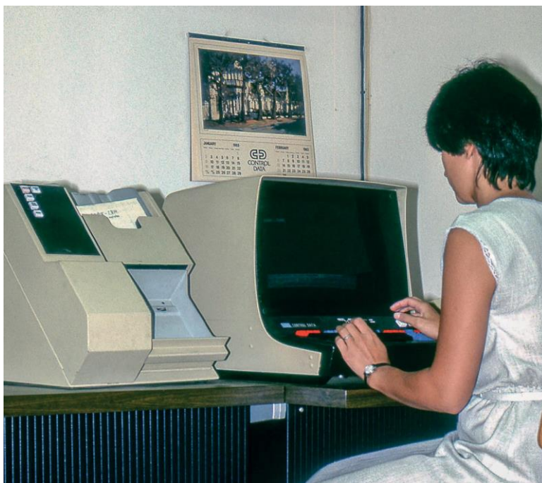
Figure 9 Mrs Anne Mans at the workstation that was connected to the CSIR's powerful computer. To her left is the punch card reader. This station also had a printer that is not visible on this photo. (Source: Photo collection of Mrs AD Mans)
